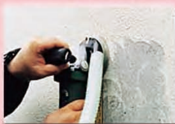
Removing elastic coating.
