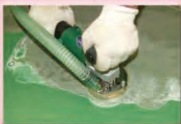
Removing epoxy coating.
