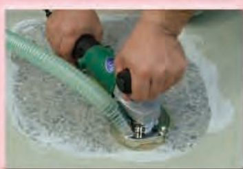
Removing urethane coating.
